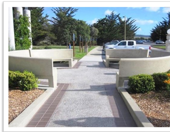
Precast Concrete Seat wall
